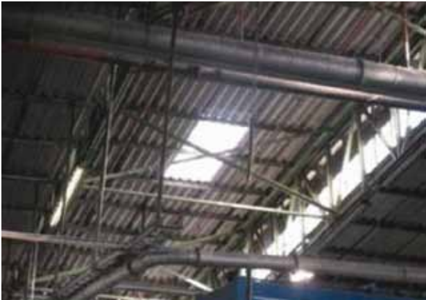
Installation of translucent roof sheets to increase sunlight into the building, thus minimising electricity usage for lighting
