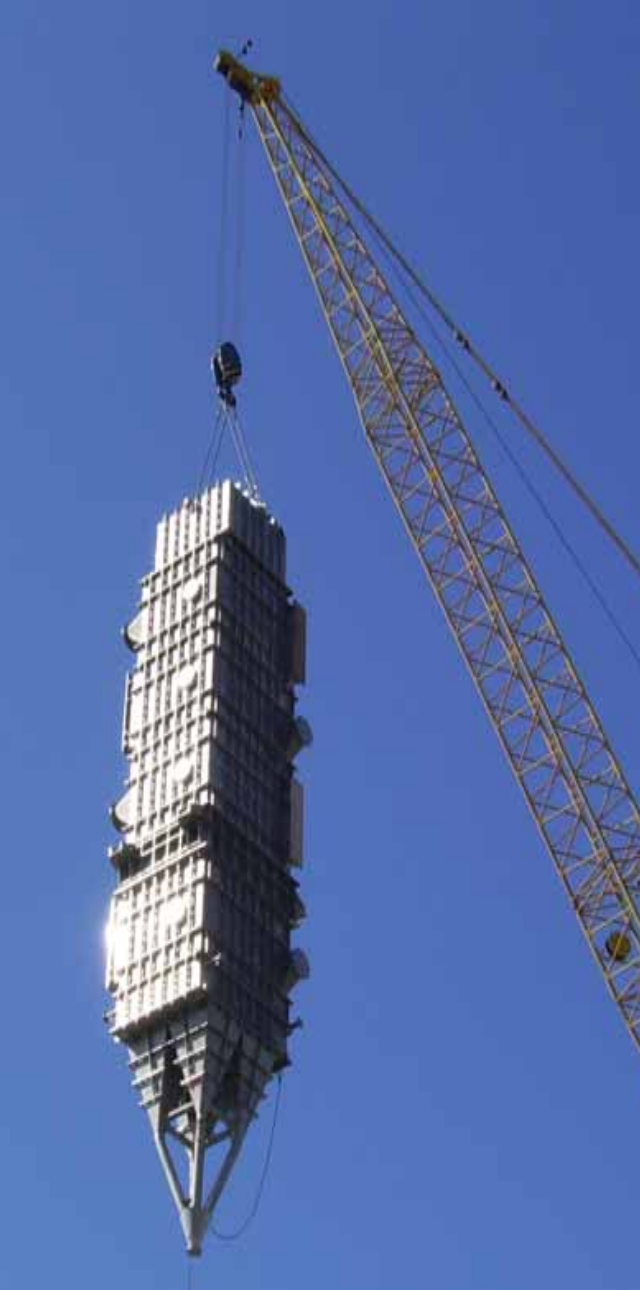
Preheater & Reactor being installed
