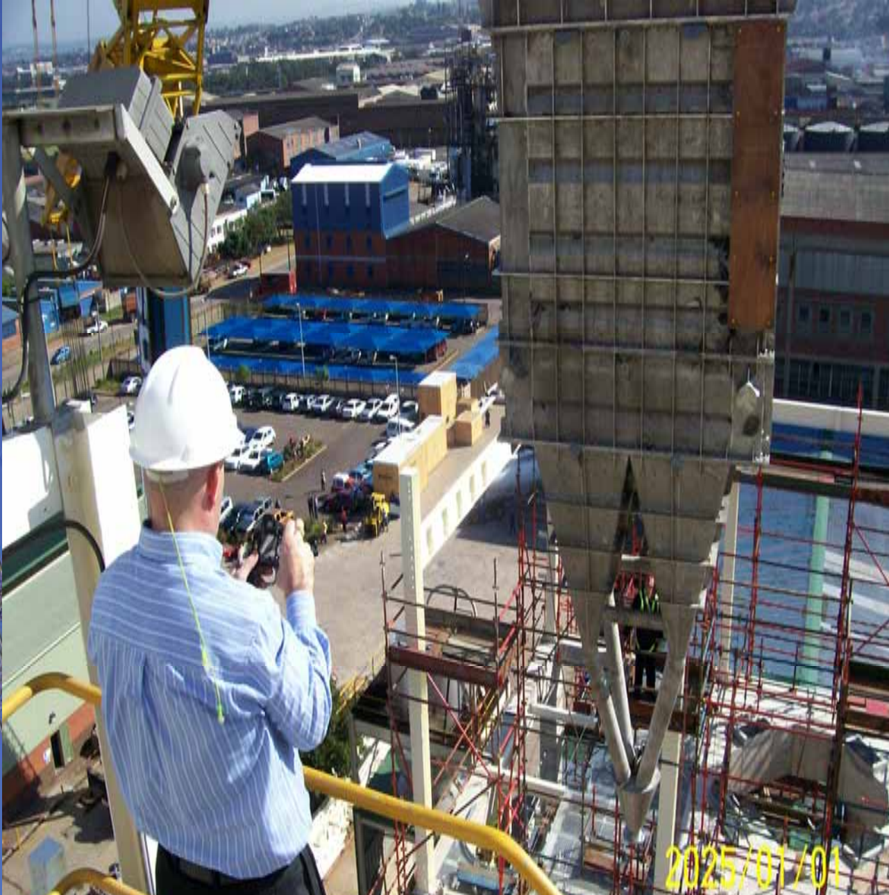
Preheater & Reactor being installed
