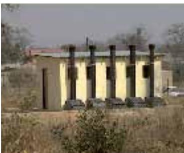
ENVIROLOO ABLUTION BLOCKS
